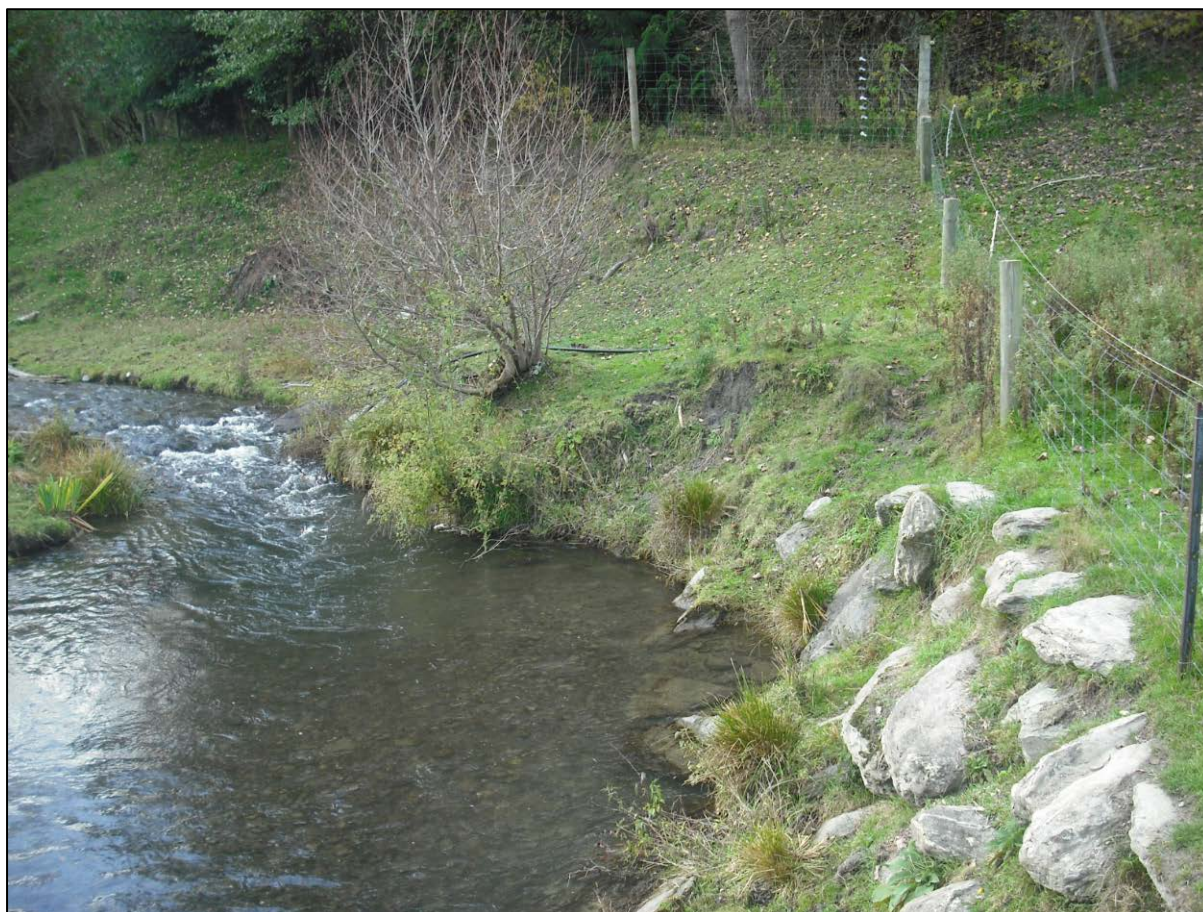
Figure 4.4: Scour Protection with Rock Structures
