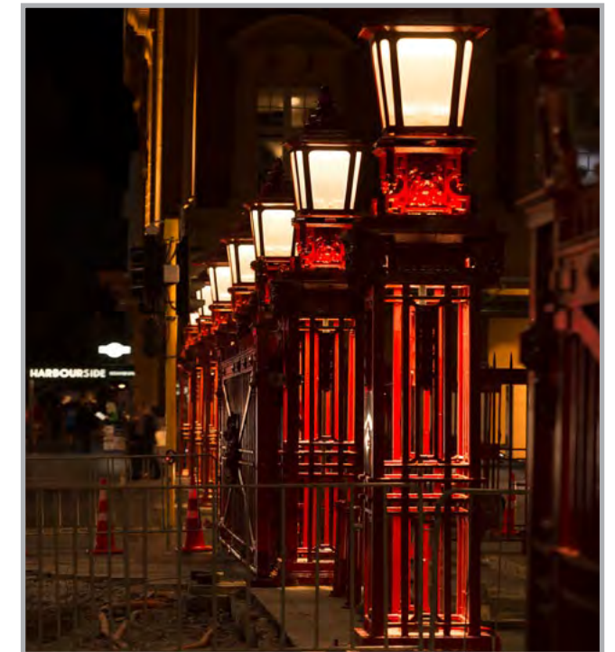
Example of traditional street lanterns refurbished with LED light source.
