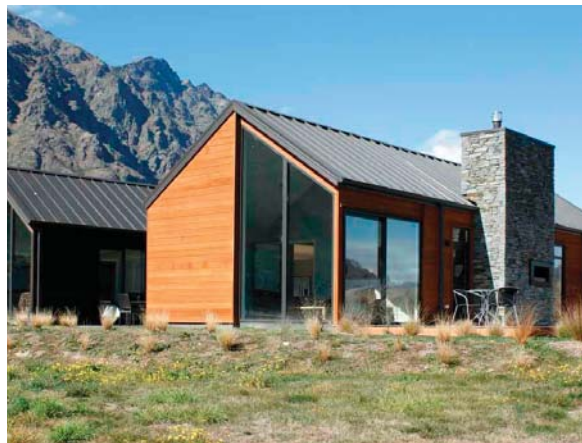
IMAGE 16: ROOF PITCH & MATERIAL
