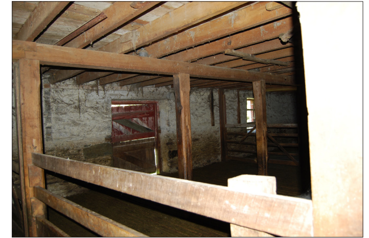
View inside original stable. Existing slatted floor and original floor level to be reinstated
