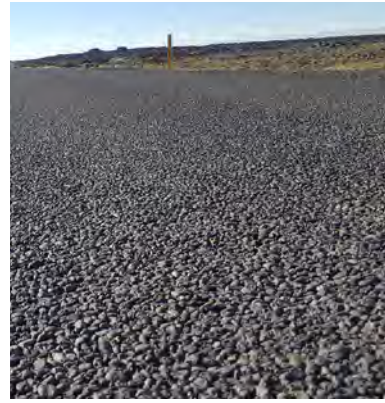
Chip Seal (Internal access)
