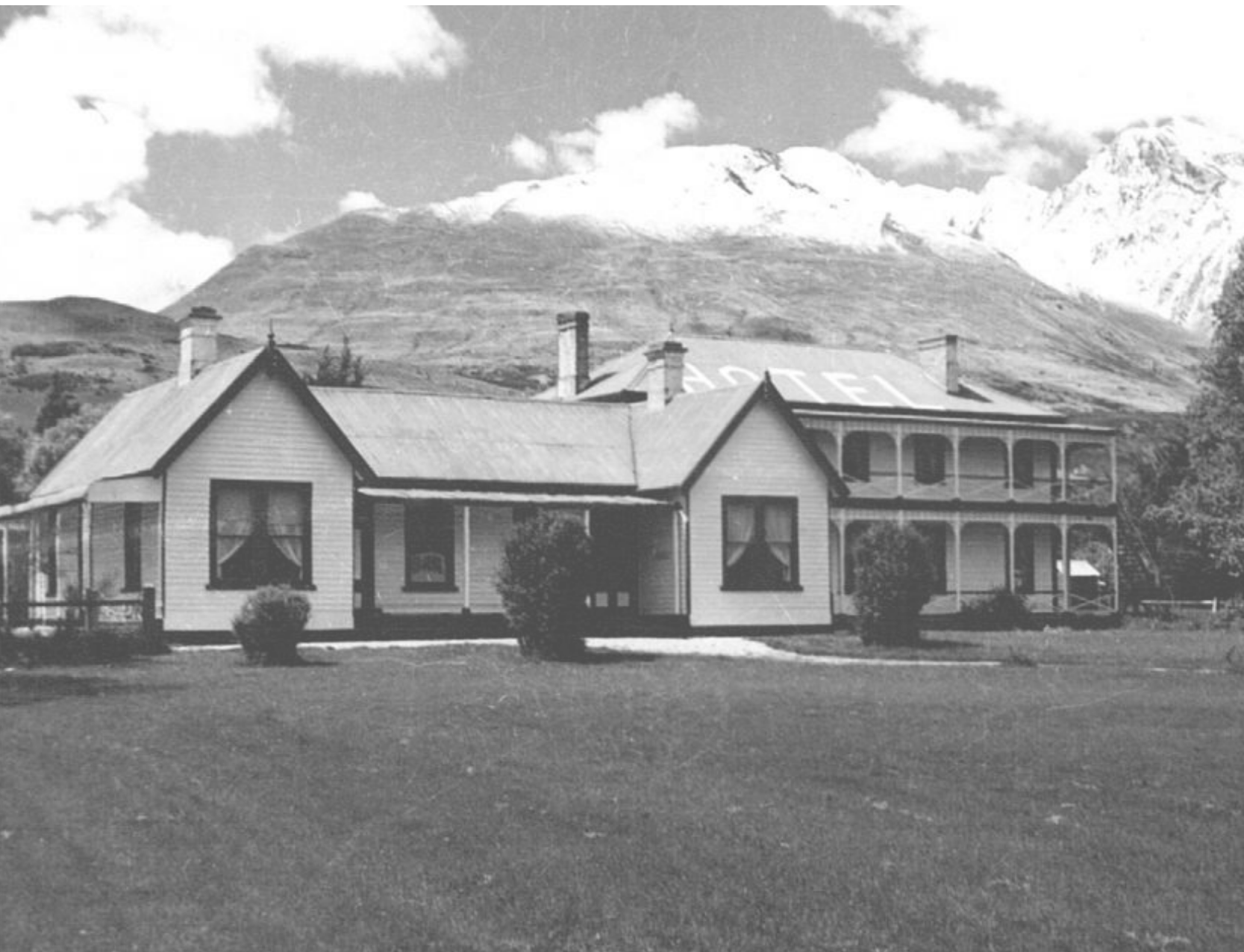
The Mt Earnslaw Hotel in 1959 prior to destruction by fire (Eric Livingstone; 1959 eHive).
