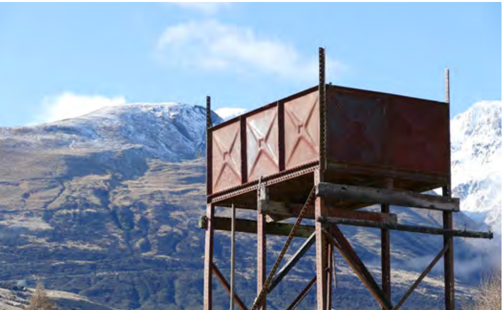
The existing tank stand, to be relocated as an entry marker
