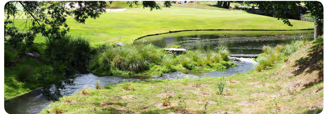
Example of creek widening and use of weirs at Millbrook Resort
