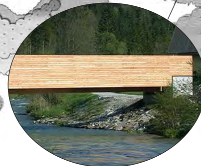
CONTEMPORARY TIMBER BRIDGE
