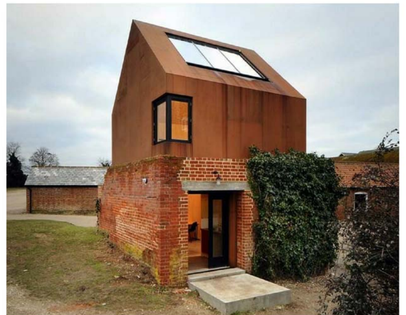
Precedent image of steel panels used in an adaptive re-use of a heritage building
