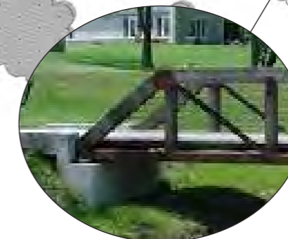
HERITAGE PEDESTRIAN ACCESSWAY
