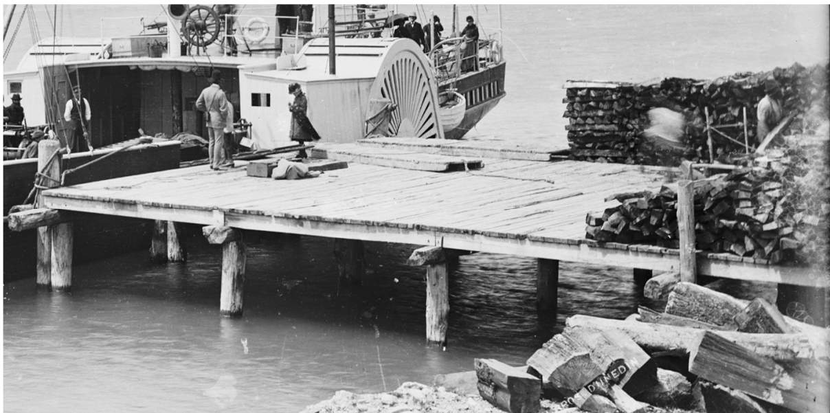
A crop of a photograph 35 taken in January 1883 of the Mountaineer at Kinloch Jetty. The jetty appears to be comprise a plain, rectangular deck, without railings, supported on 3 rows of single piles and a double row closest to the ship.
