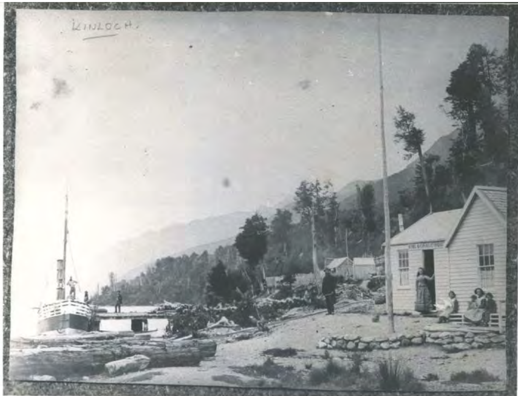
Kinloch, Wakatipu 21 – this photograph is undated but is likely to date from the early to mid 1870s. The name of the building above the doors indicates that this is the Kinloch Accommodation House.
