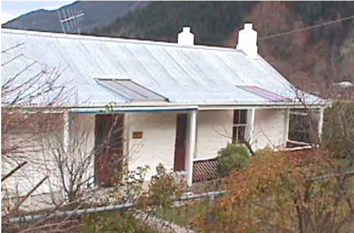
Thompson House 66 Hallenstein Street, Queenstown
