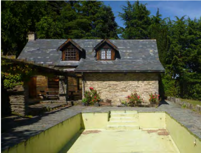
Condition of The Loose Box as of December 2013
