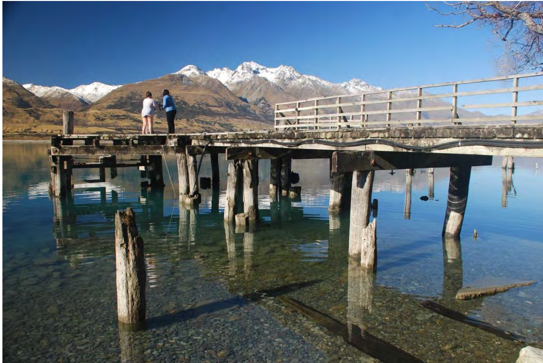
The northside of the jetty today; the post in the foreground indicates its former width with the gap between it and the people being where the wharf building once stood (it is now on the shore adjacent). Truncated posts sticking up just above lake level appear to be the remains of the first jetty on the site.
