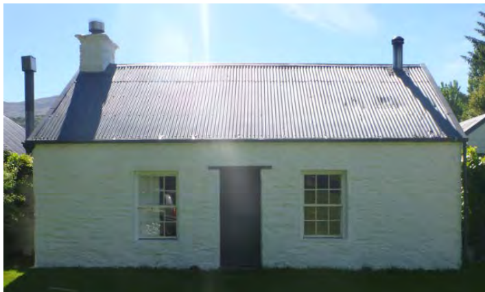
McMaster House (original part), December 2013
