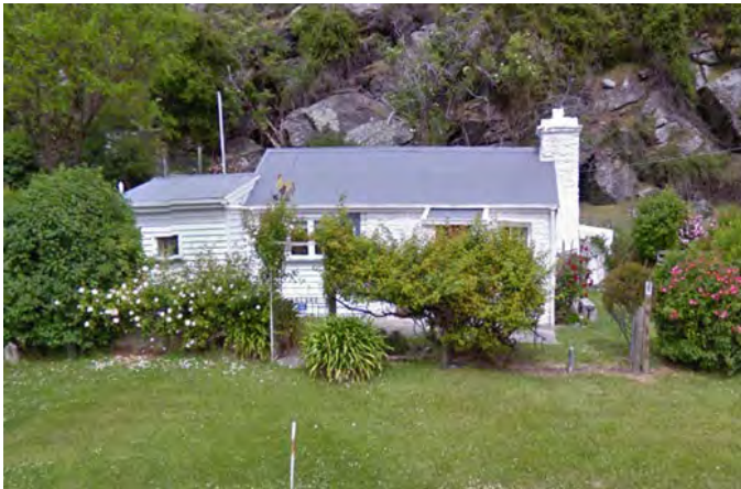
148 Kingston Road, Google Earth, December 2013
