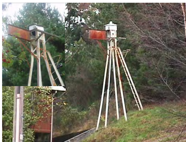
Former One mile leading light, near YHA, Esplanade
