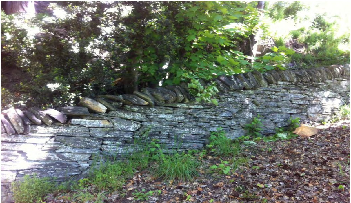
Image Three: Stacked schist along the top (Inano Walter, 2013)
