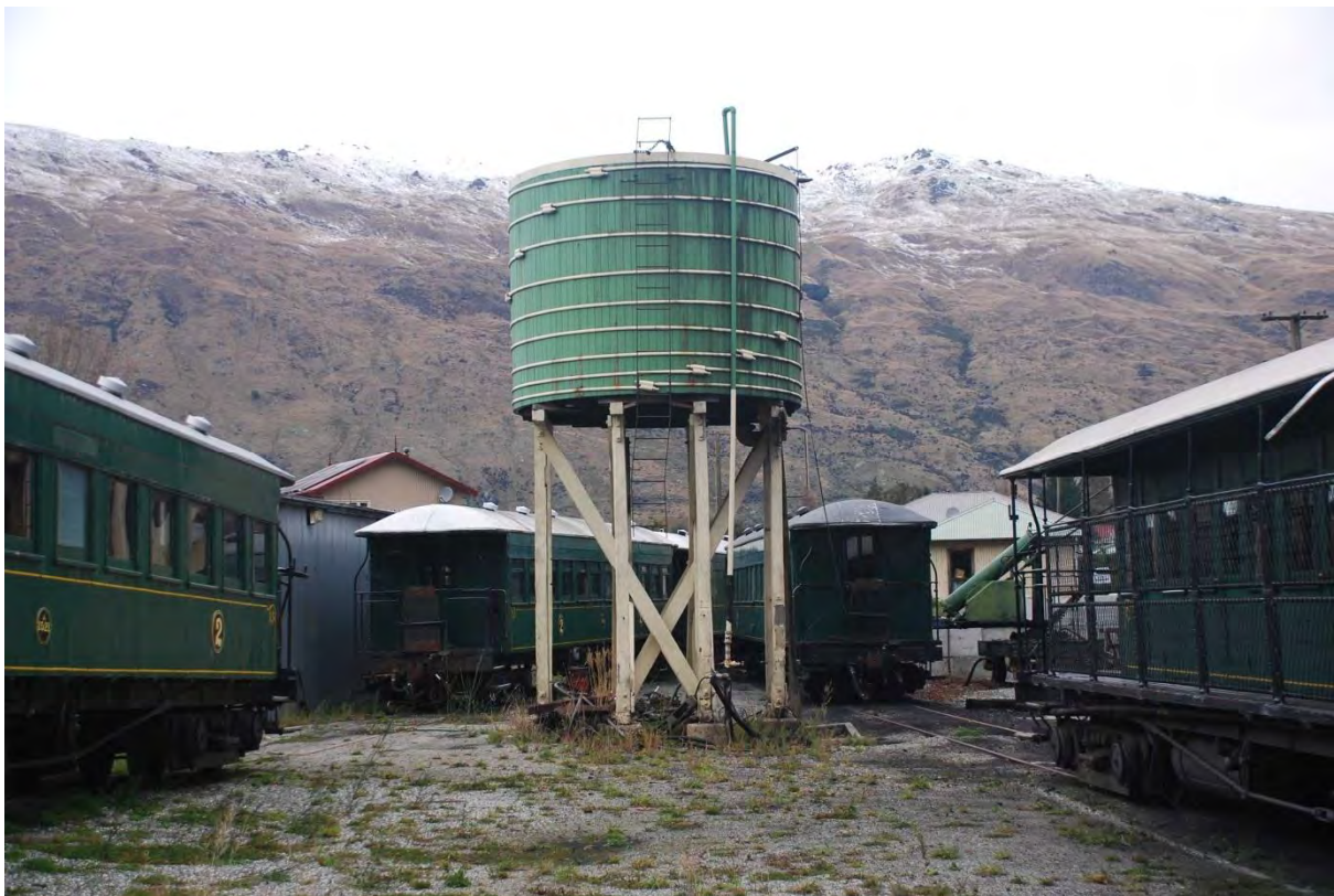
Photo 2 The water tank in the Kingston station yard/depot
