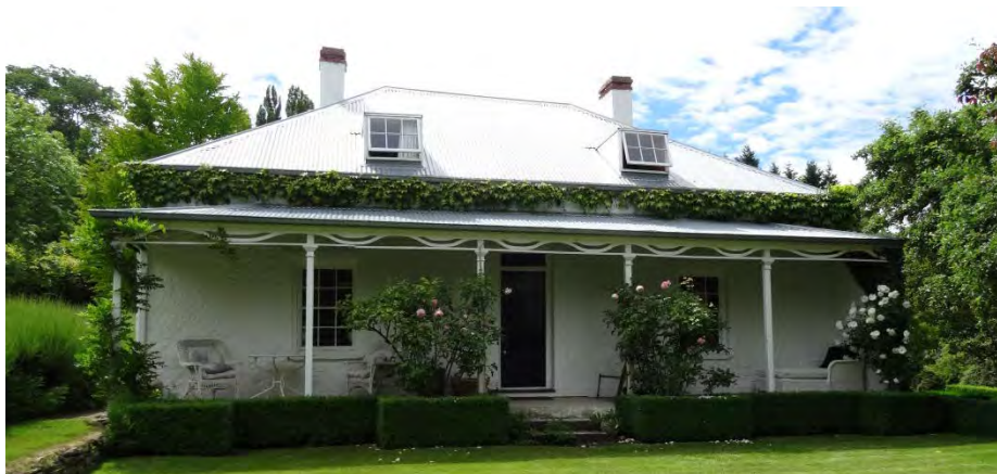
Front of house, December 2013
