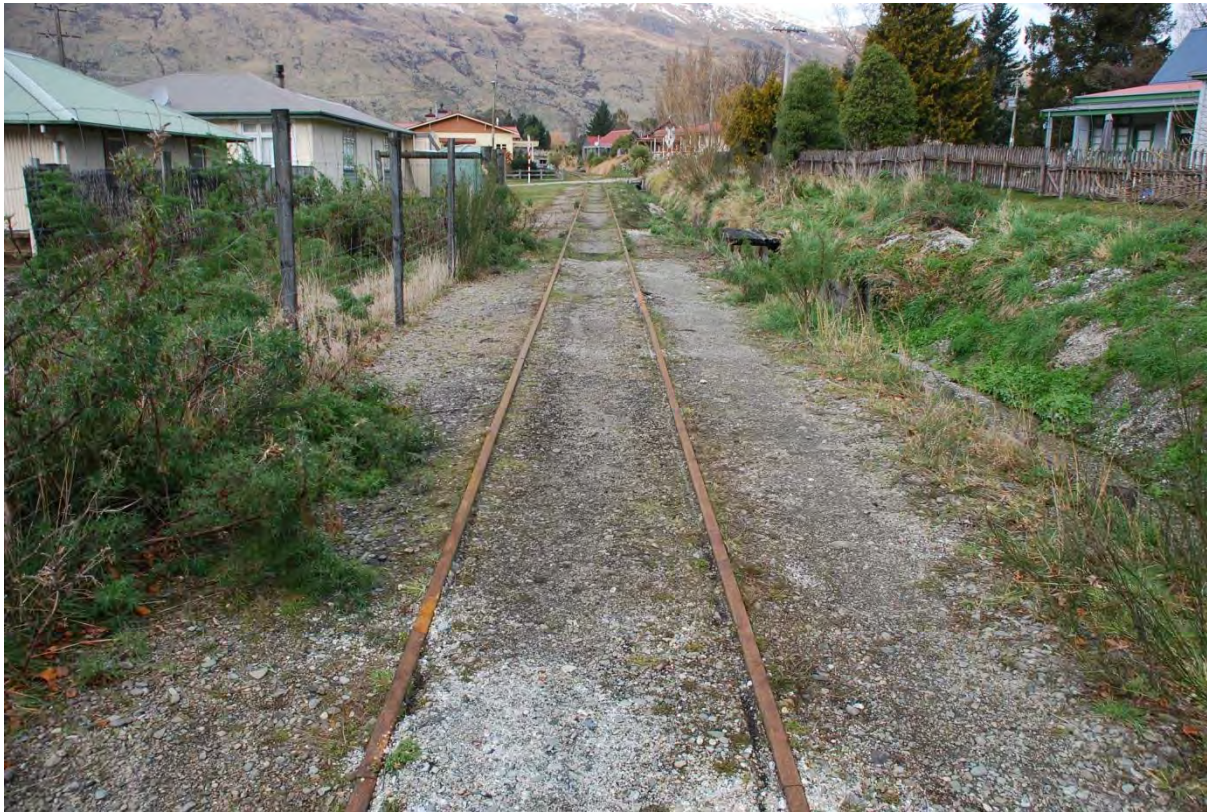
Photo 1 The railway lines adjacent to Kingston station yard/depot
