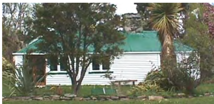
North elevation (older portion of Ship Inn)
