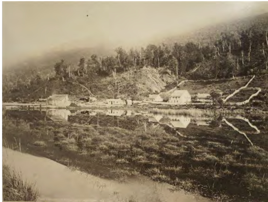
Kinloch, circa 1870's. Shows Kinloch lodge central building with two accommodation lodges either side. (EL 4203 in EA37 LDM)
