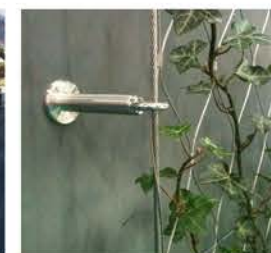
Climber planting on wire structure to building facade of hotel and for buttresses
