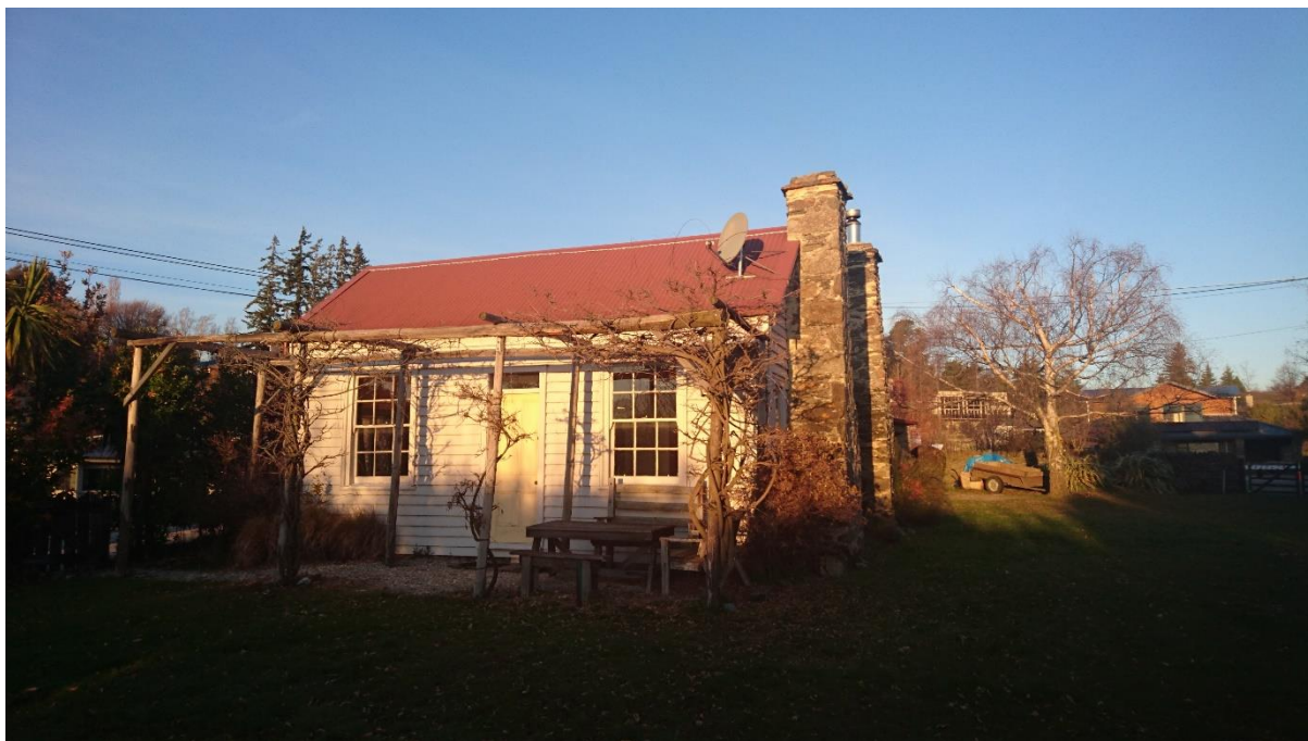
Photo 3 North elevation – Origin Consultants 28 June 2019
