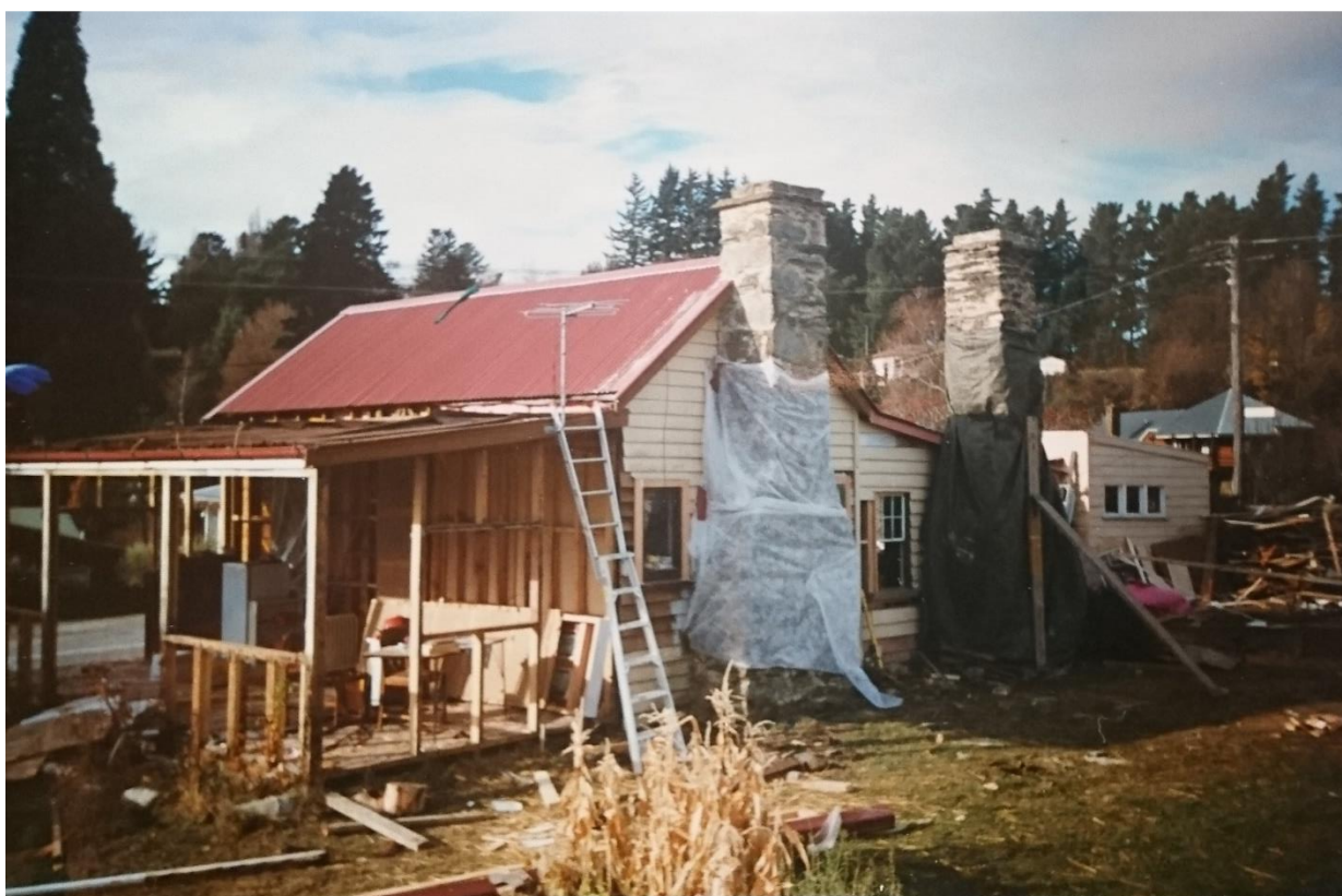
Photo 6 Refurbishment c. 1994 – photo supplied by present owners
