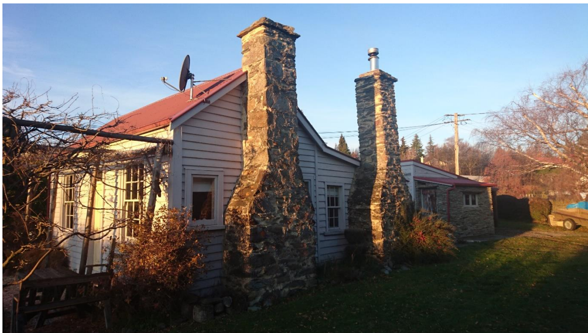
Photo 4 West elevation – Origin Consultants 28 June 2019
