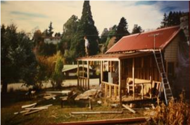
Figure 6: Removal of addition at the front of the cottage (Eliott collection)
