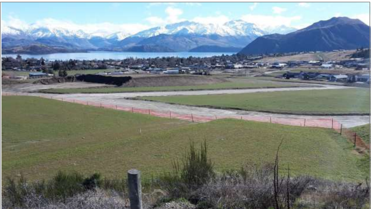
Figure 5: Unstabilised topsoil stockpile
