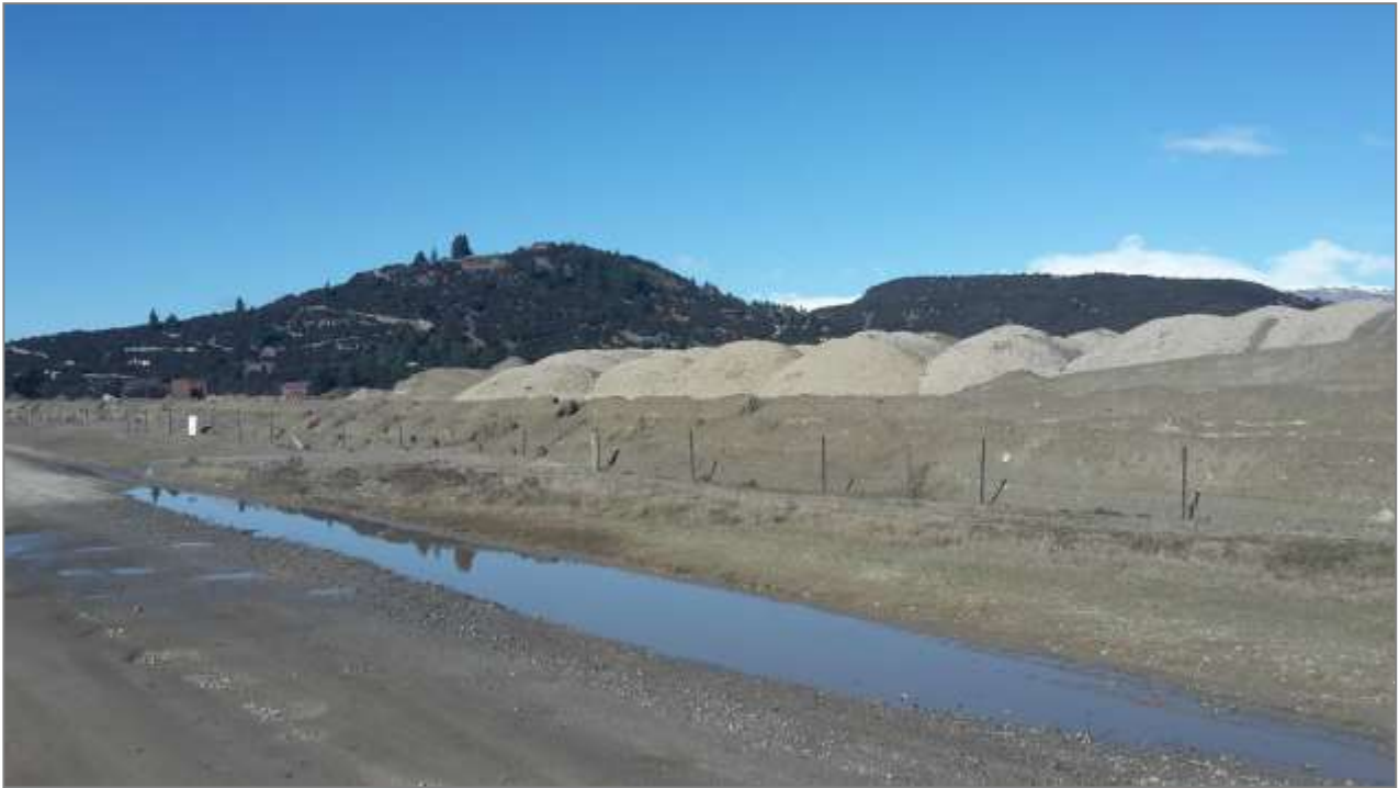
Figure 1: Topsoil stockpiles with no sediment control
