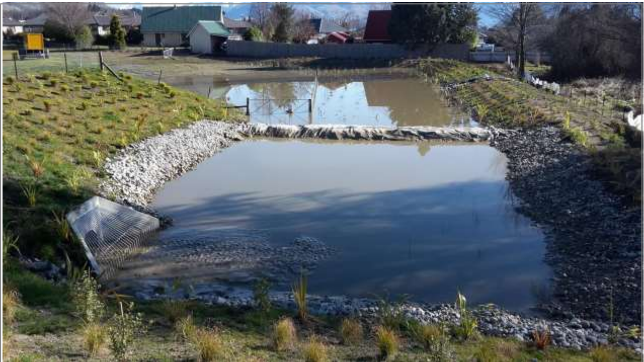
Figure 7: Sediment collected in a completed stormwater pond from Figure 6 catchment (the stormwater pipe was half full of sediment and will require extensive mucking out)
