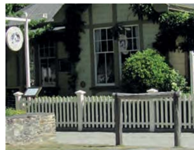
Traditional picket fencing fronting the Postmasters Restaurant, Buckingham Street.
