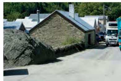
Photo looking east along Arrow Lane showing the dominance of the shed form and extensive variation of building setbacks off the Lane.
