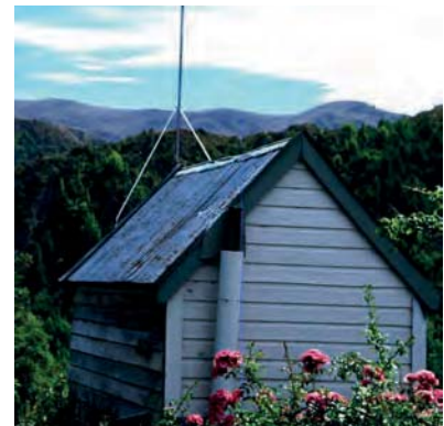
Small shed-out building.
