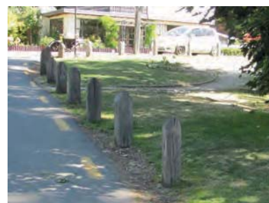
Good example of simple timber bollard.
