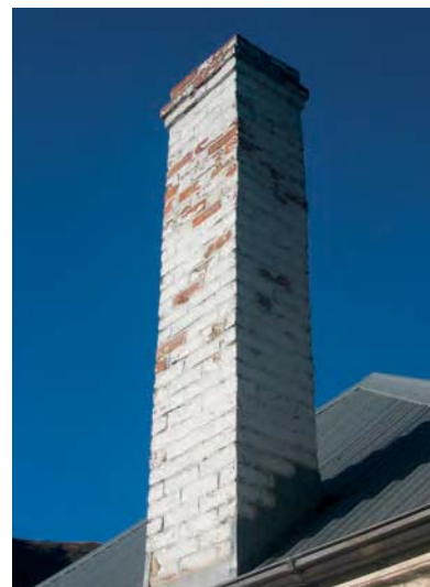
Use of brick limited to chimneys and trim.
