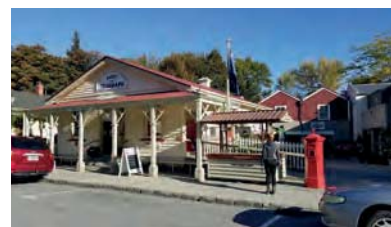
Open Space area to the north west side of Post Office, which is now integrated with the Post Office Precinct development to the rear.
