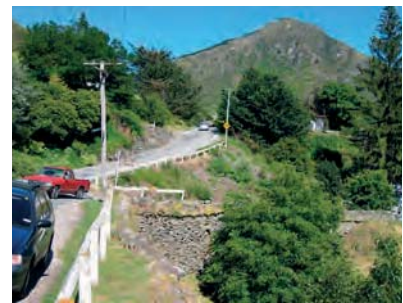
Butlers wall, Villiers Street behind.
