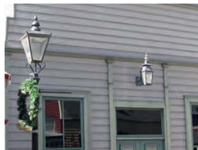
Appropriate style streetlighting, linking with exterior façade lighting.
