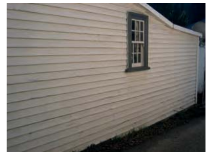
Painted Weatherboard with boxed corner.
