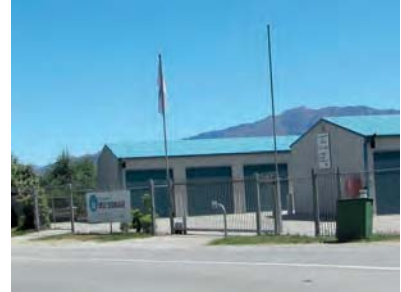
View of Industrial storage units viewed from Manse Road.
