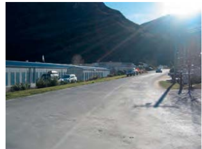
View of Industrial storage units looking north from Manse Road.
