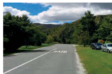
Narrow carriageway gravel shoulders, grass swales and verges with street trees.
