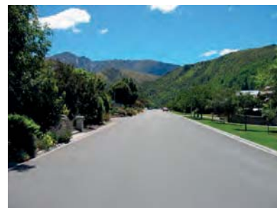
Avoid excessively wide carriageway with low profile kerb and channel.
