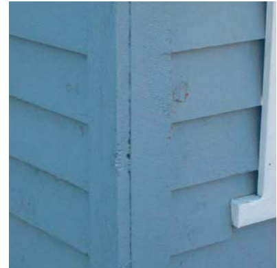
Painted Weatherboard with boxed corner.
