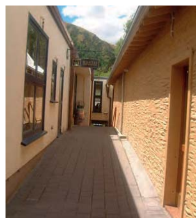
Uninteresting pedestrian link with poor detailing.
