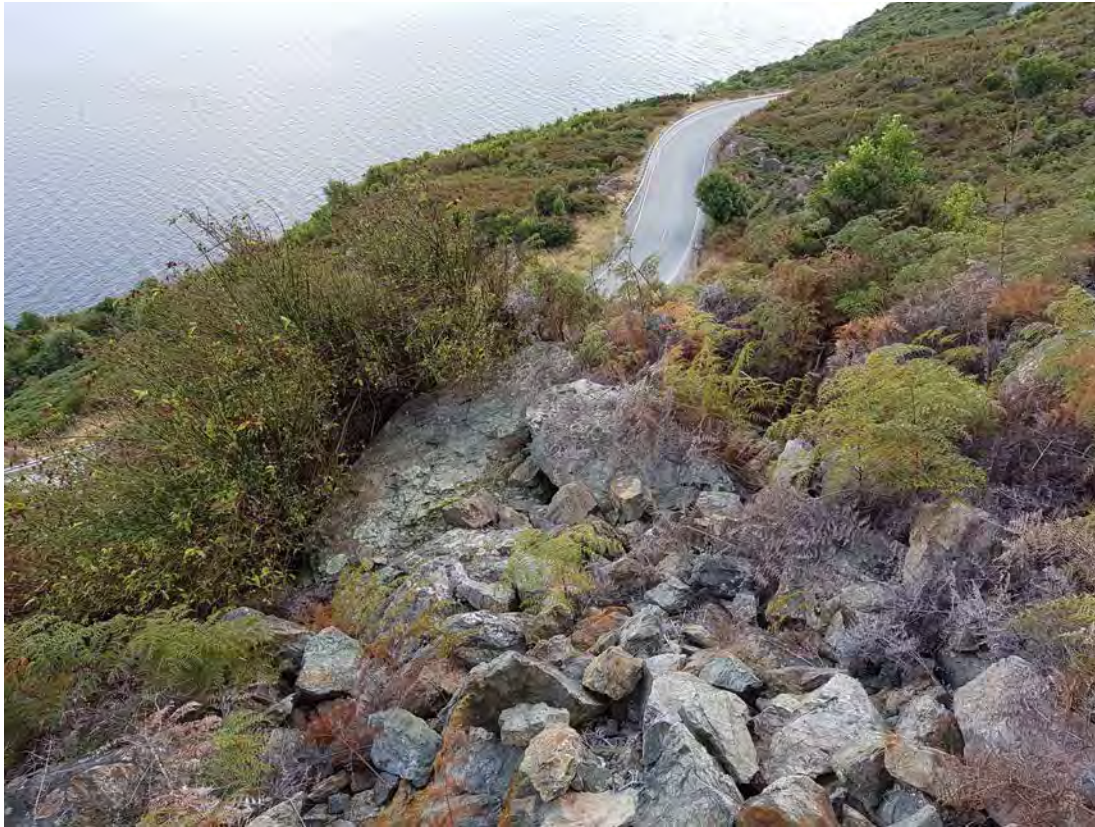
Photograph 2.1 – Showing the rock fall debris on the slopes above the road and below the main tension crack and monitoring locations.
