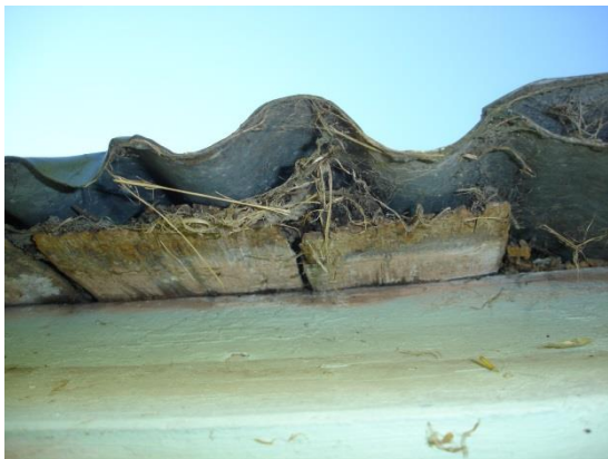
Detail of timber shingles visible under the corrugated iron at the eaves.
