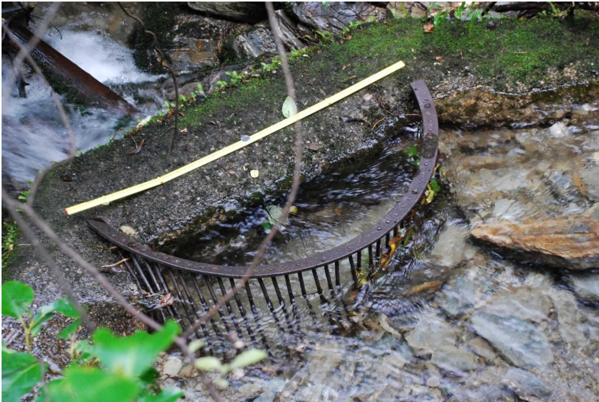
Photo 2 The half-round iron grill protecting the mouth of the supply pipe at the weir (with yellow 1000mm rule).
