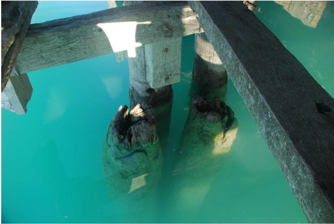
The remains of doubled-up piles probably dating to the first jetty of c.1873.
