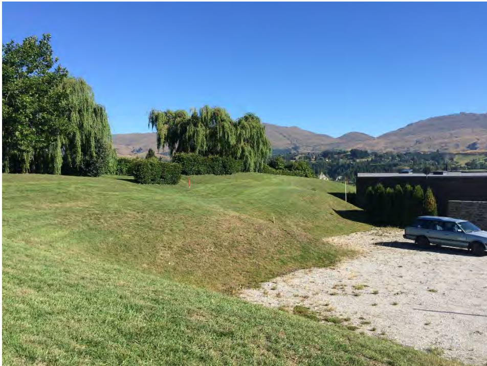
Photograph 4. Looking North West at the Building Extension and Earthworks Area. Source – Sean Dent 26.02.15
