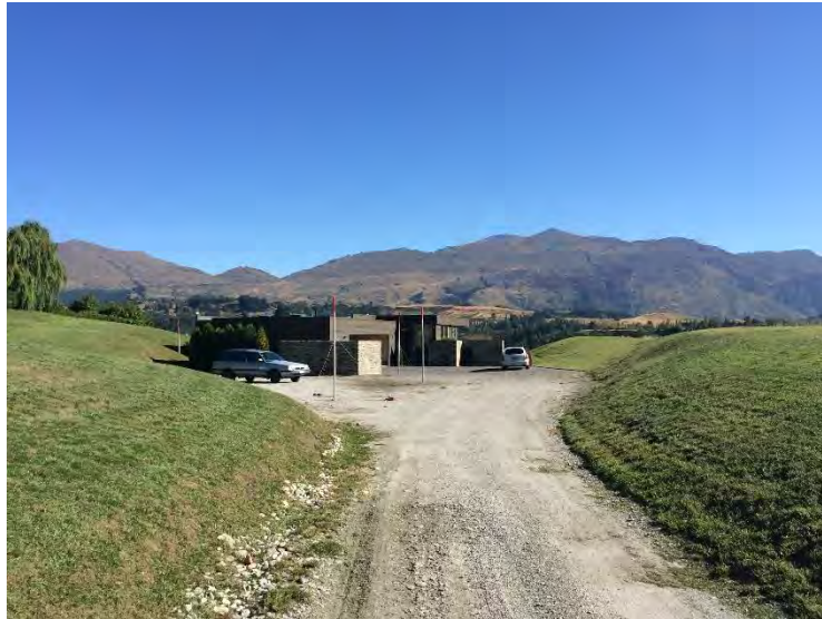
Photograph 2. View of Access Way and Mounding taken near the South Eastern corner of the Subject Site. Source – Sean Dent 26.02.15
