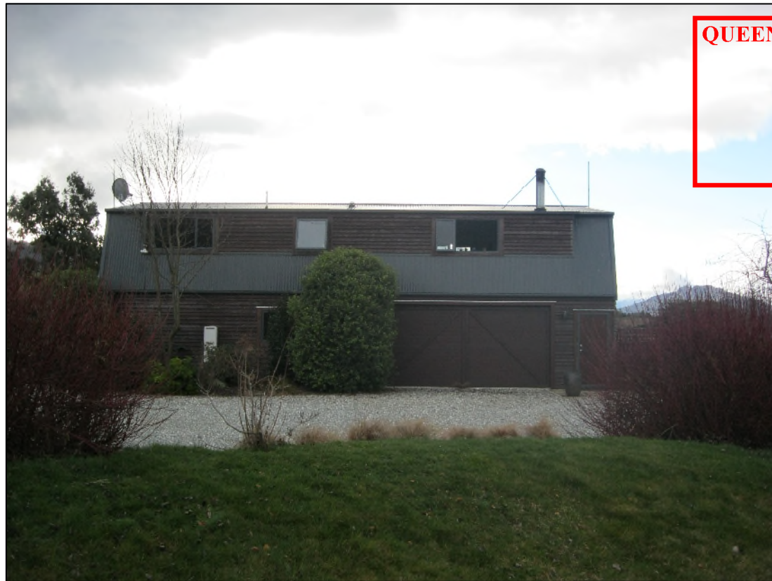
Existing House from the South 22/08/13
