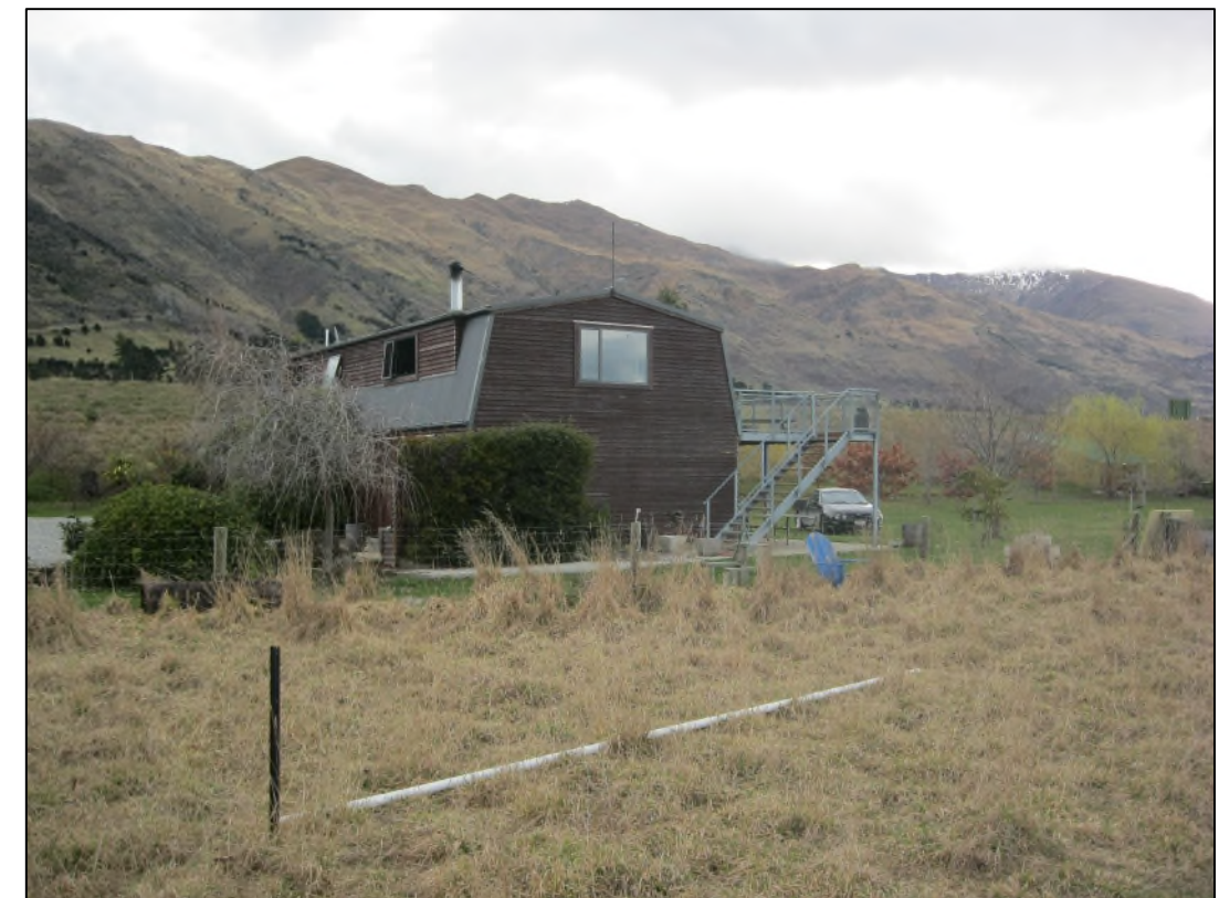
Existing House from the East 22/08/13
