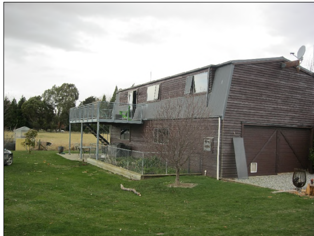
Existing House from the North 22/08/13
