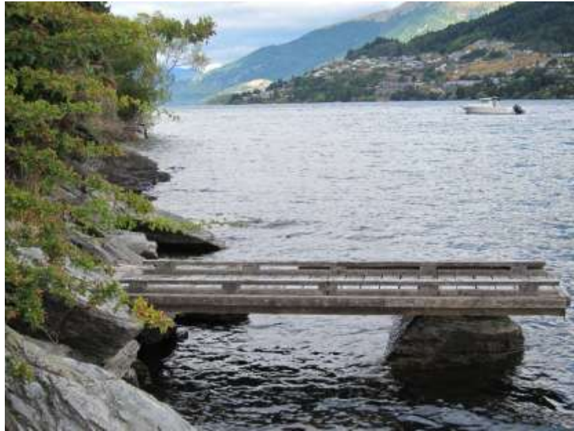
Existing jetty east of the proposed jetty location
