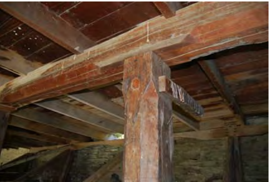
Timber post and beam with floor joists and flooring retained
