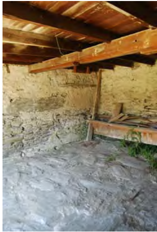
Re-instate window and fireplace shown enclosed. Flagstone floor to be displayed with glass floor over in selected areas.
