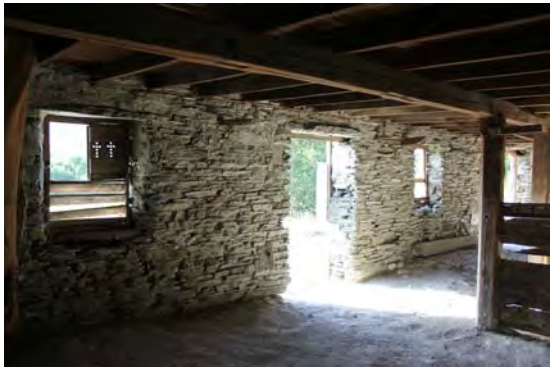
Retain existing opening and window treatments. New windows and doors to be positioned on the interior side.
