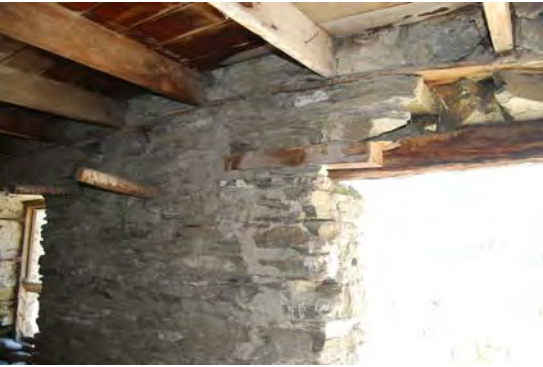
Saddle rails retained where possible and used as towel/robe hooks
