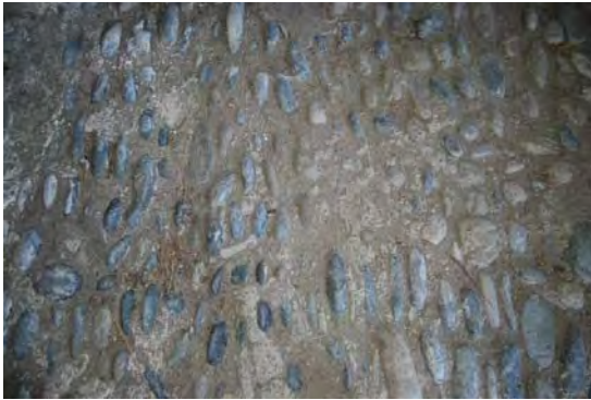
Cobbled stone floor retained and displayed in selected areas with a glass floor over
