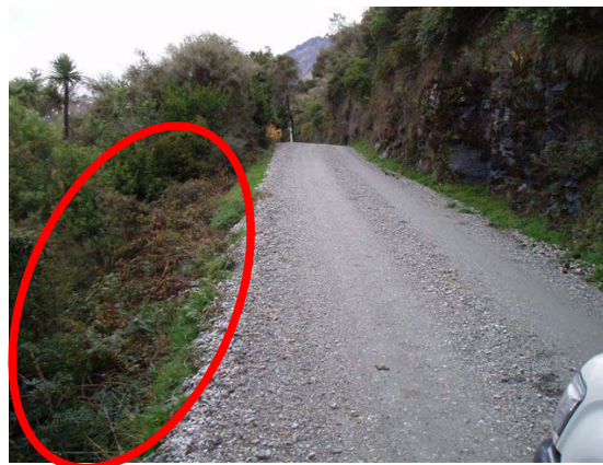
Figure 14: Imprint of Straying Vehicle on Roadside Scrub
