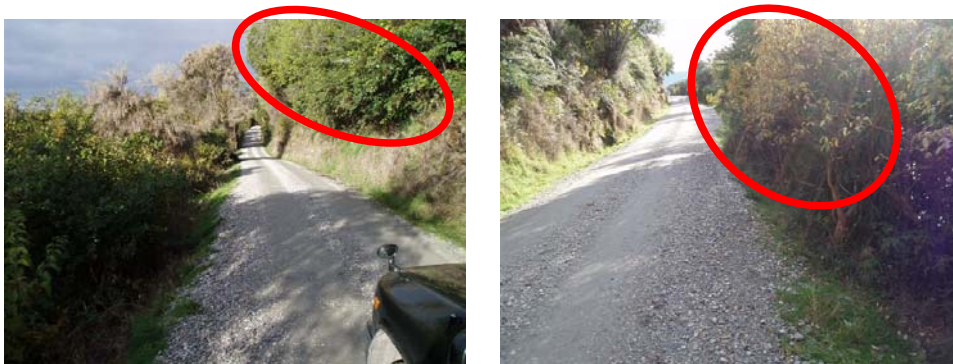
Figure 13: Encroaching Brush on Sides of Road
