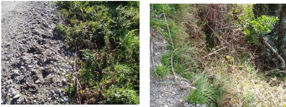
Figure 16: Unsupported Metal at Road Lakeside Edge
