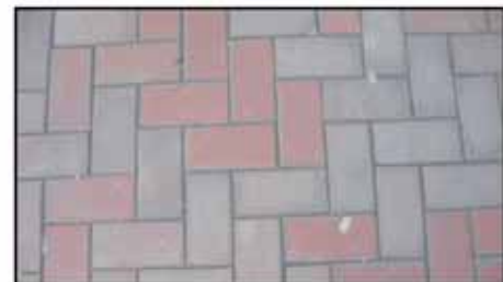
Modern coloured tiles are inappropriate to historic character
