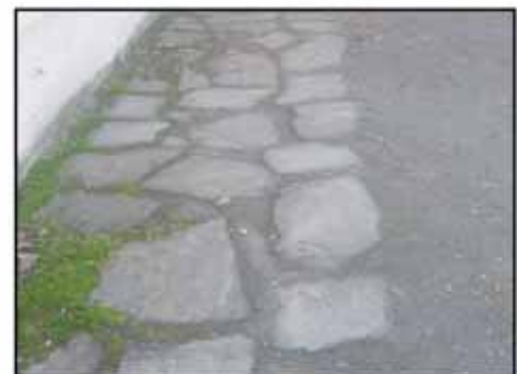
Stone set in crusher dust and gravel path.
