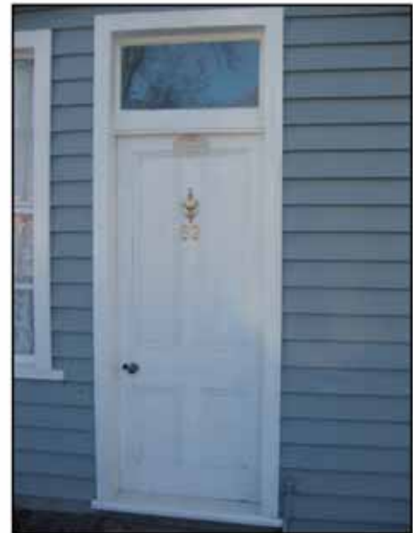
Frame and panel door with top light
