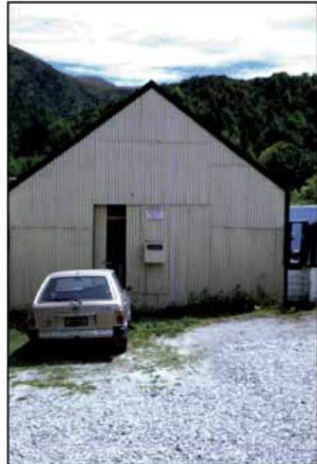
The simple back of a false front shop primary element as seen from the Lane.
