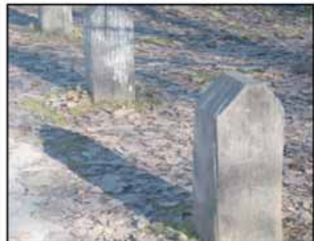
Simple timber bollard.
