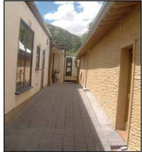
Uninteresting pedestrian link with poor detailing.
