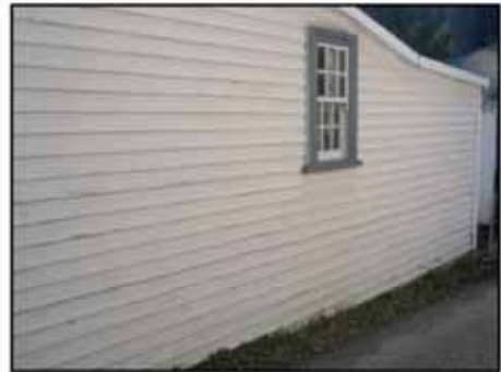
Painted weatherboards with boxed corner
