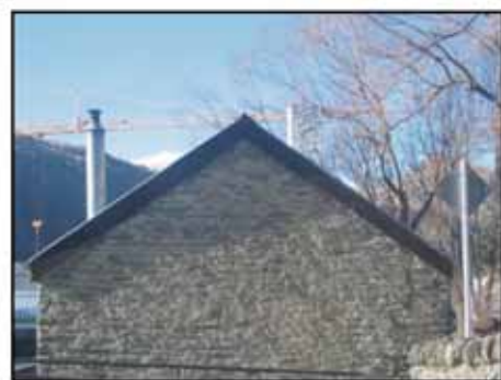
The simple form of the shed.
