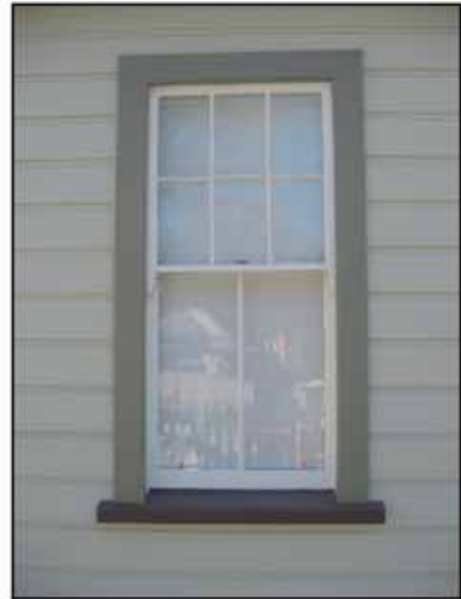
Window -double hung with lattice. Double-hung window
