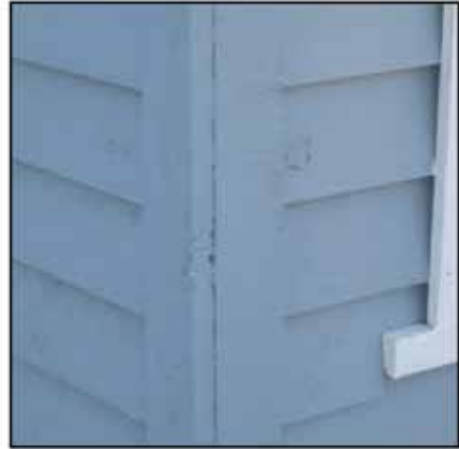
Painted weatherboards with boxed corner
