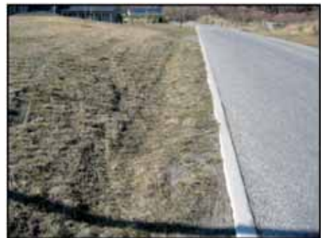
X Grass drainage swale and flush concrete edge to seal. Instead place concrete beneath seal edge.
