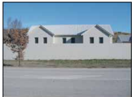
Masonry walls-complete fortification
