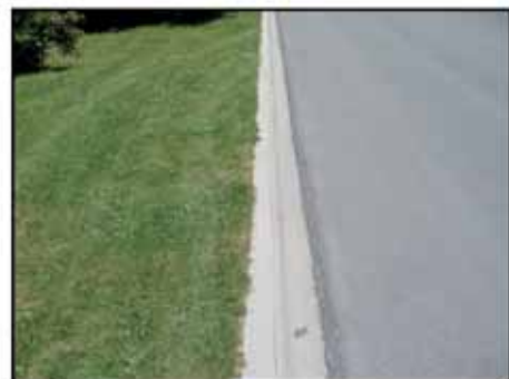
Low profile kerb and channel.
