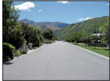
X Excessively wide carriageway with low profile kerb and channel.
