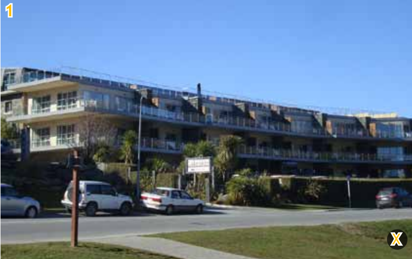
Excessive repetition of units
