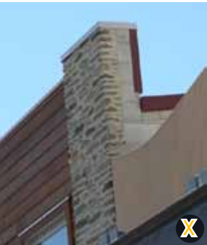
Parapet detail exposed
