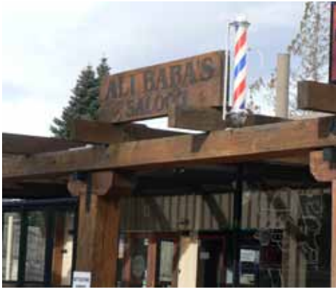
Large exposed timber members
