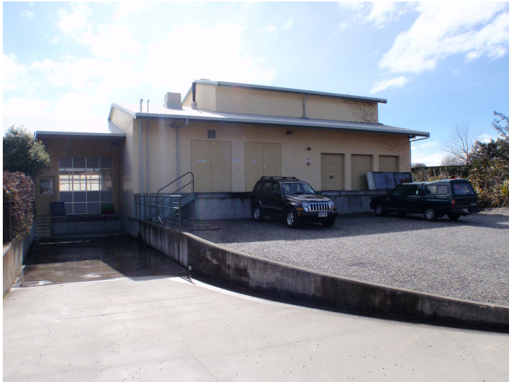
Figure 1 LDH Energy Centre
